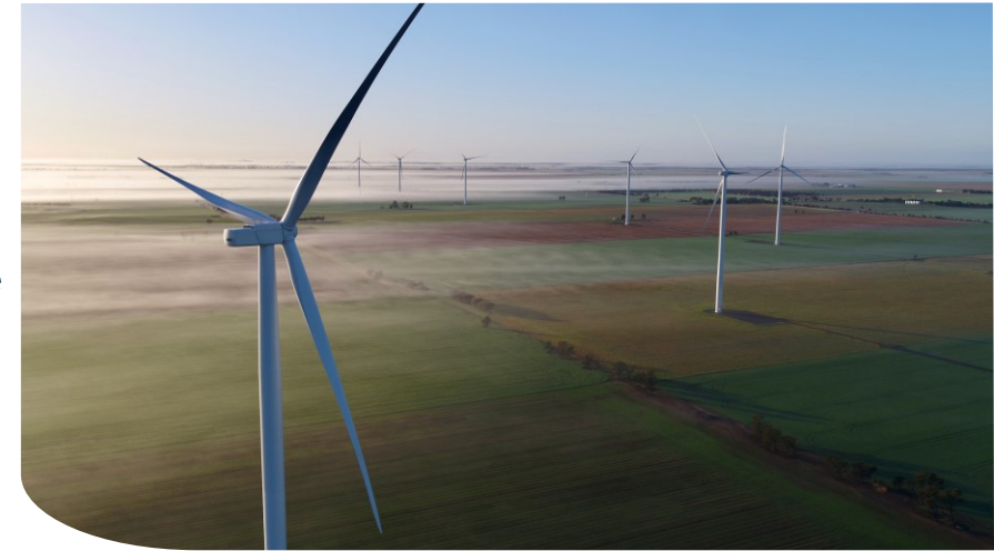
Photo: Murra Warra Wind Farm, VIC. © Squadron Energy
