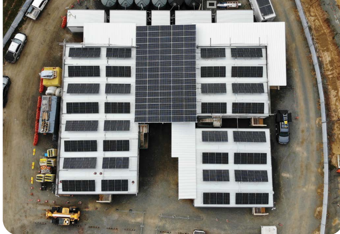
Princes Highway East Kilmany Solar, Victoria.
