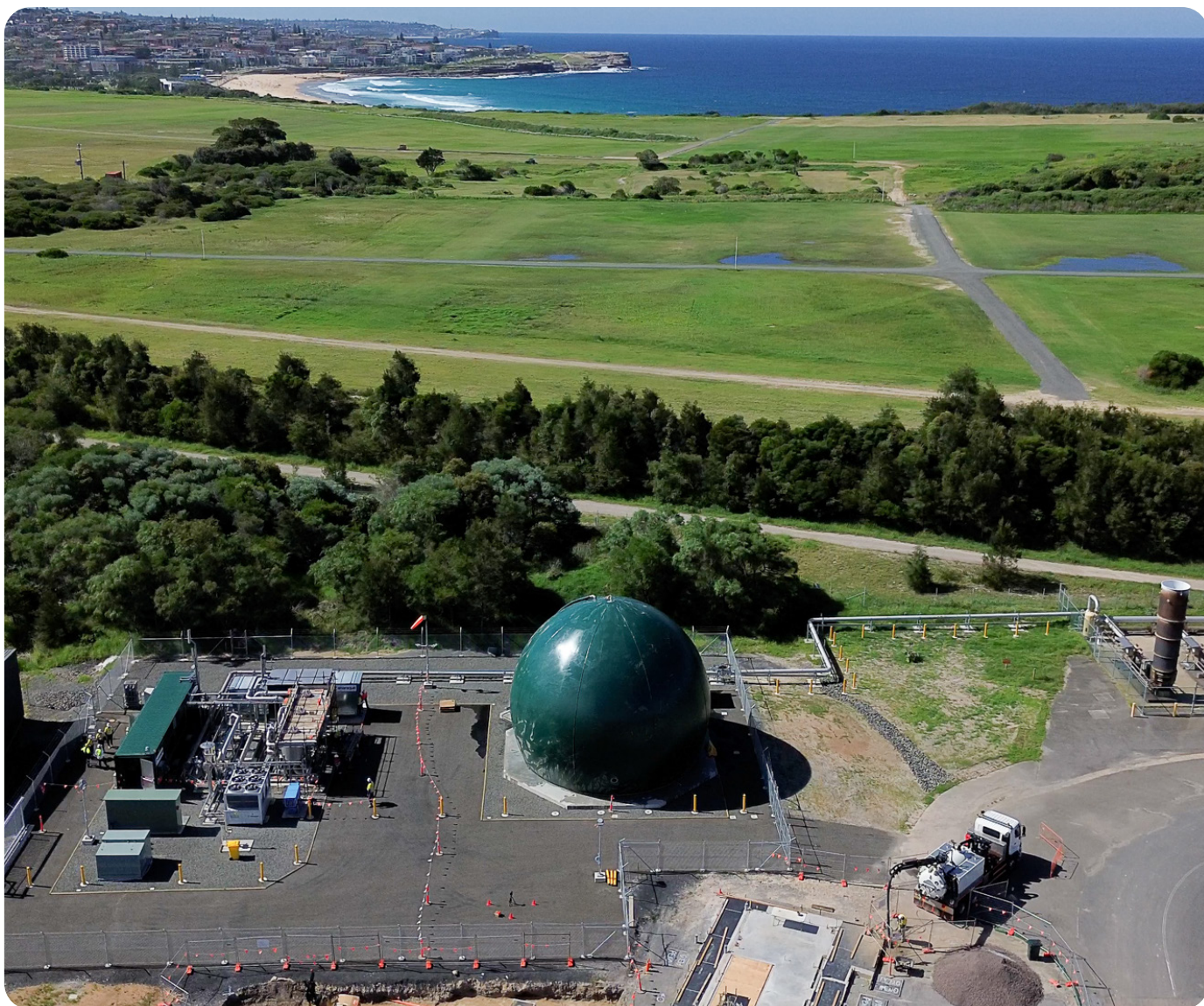
Jemena Biomethane Injection Project.
